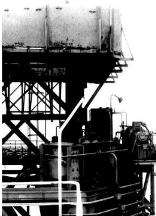
Work platforms installed
