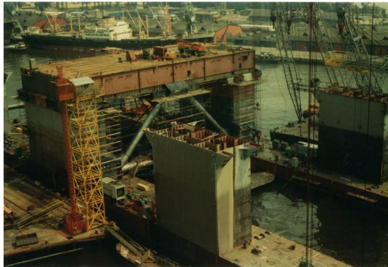
Figure 18 Columns set using floating sheerlegs (GustoMSC)
