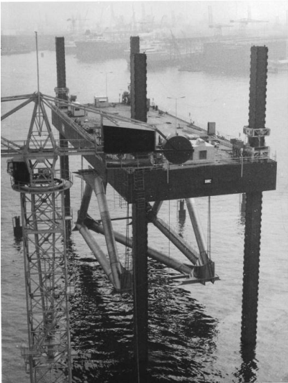
Figure 8 Setting a brace assembly (GustoMSC)
