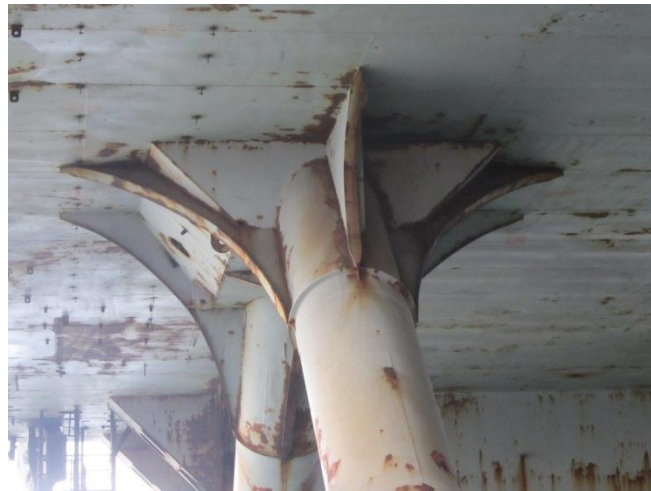
Figure 15 Brace top box in 2012 (Bart Boon)
