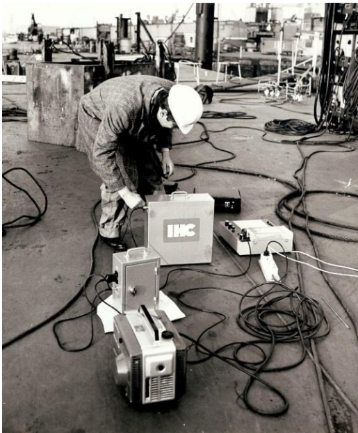
Figure 40 Measuring the heel caused by the column set-down
