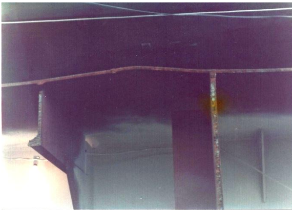
Figure 36 Buckle in block 69
