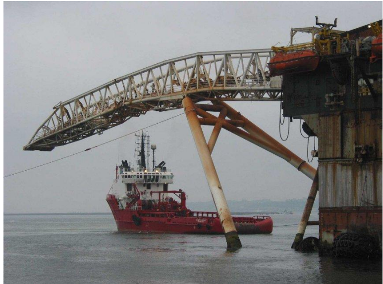
Figure 23 Stern Ramp elevated
