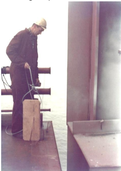
Figure 34 Wood buffer block to prevent damage
