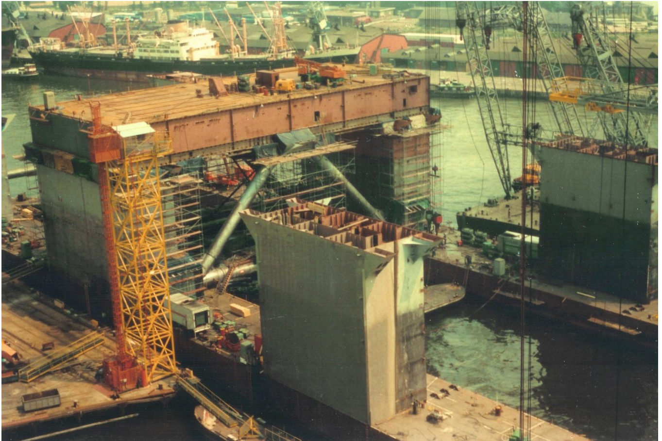
Figure 5 Floaters, columns, bracings and upper deck section
