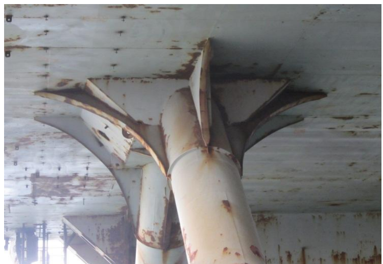
Figure 16 Brace top box in 2012 (Bart Boon)
