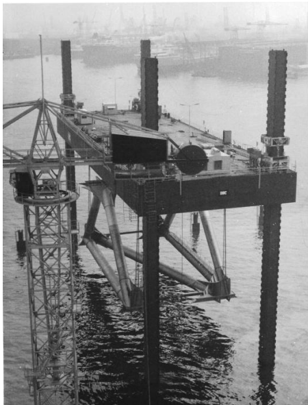
Figure 10 Setting a bracing assembly
