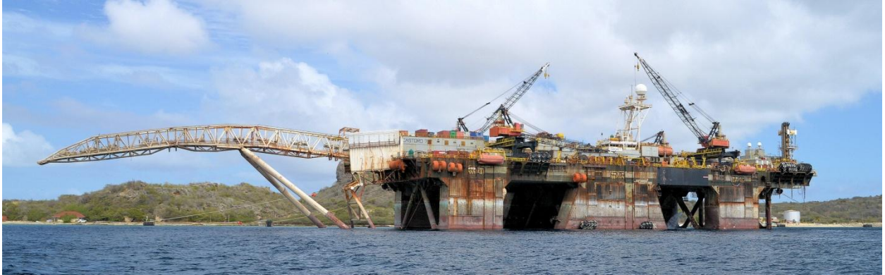
Figure 24 Castoro 7; mark the mid column modification
